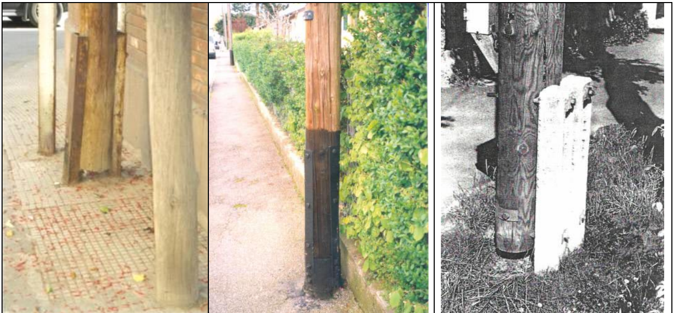
Metallic and concrete foundations
